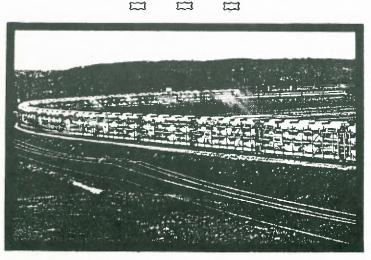
On June 9, 1959, the first Frisco piggybacked auto shipment left the Chrysler Assembly Plant at Valley Park, MO on its way to various Texas destinations. After three years of intense research and testing, the Frisco became one of the first railroads in the country to ship autos by piggyback auto carrier equipment.
