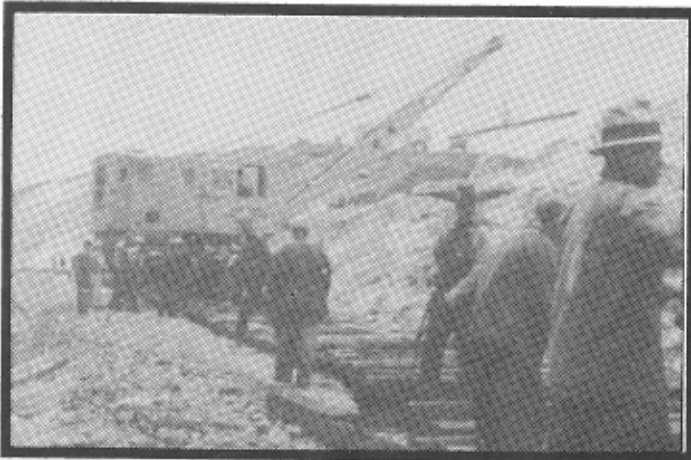
A section of the 110-pound rail being swung into position... 39 feet long, that rail weighs more than 1,400 pounds... in the foreground ties are being placed in position.
