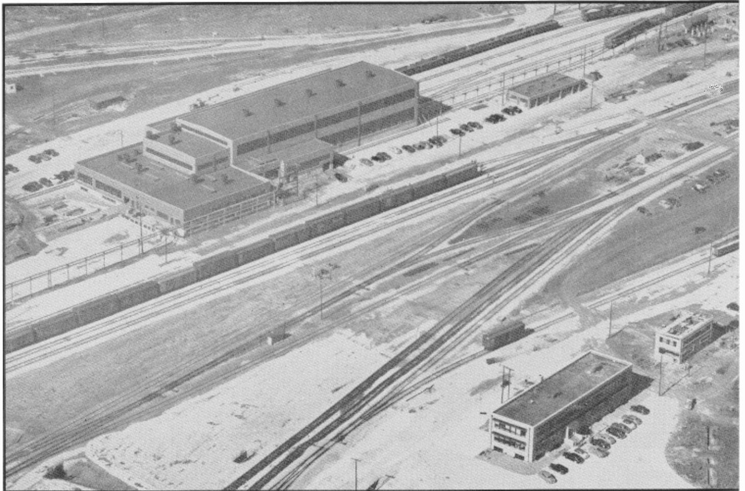
This aerial view of the Frisco's new terminal facilities at Springfield was featured in the 1949 company annual report and included a view of the new diesel shops, yard office, and restaurant (to the east of the yard office). Only the diesel shop and yard office remain today. Frisco photo
