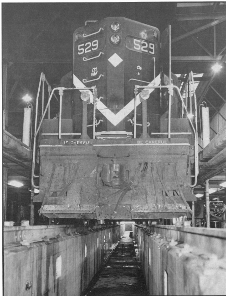
View from inside the pit area under one of the three elevated service tracks Frisco photo
