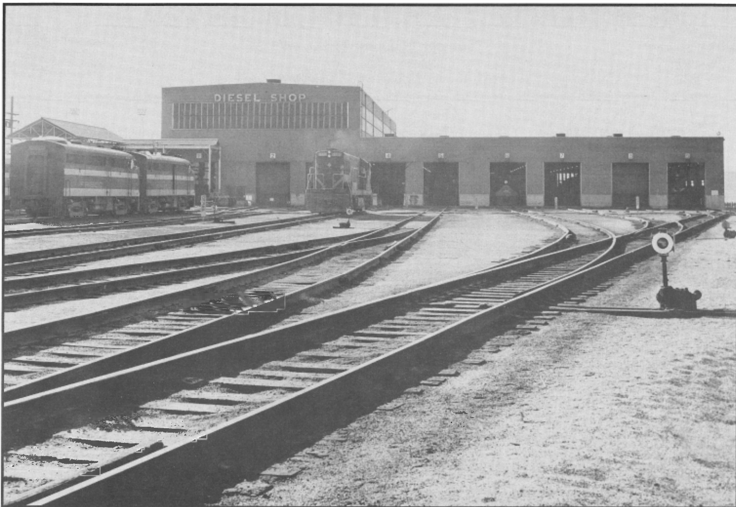
East end of diesel shops showing completed four stall extension on the north side. Frisco photo
