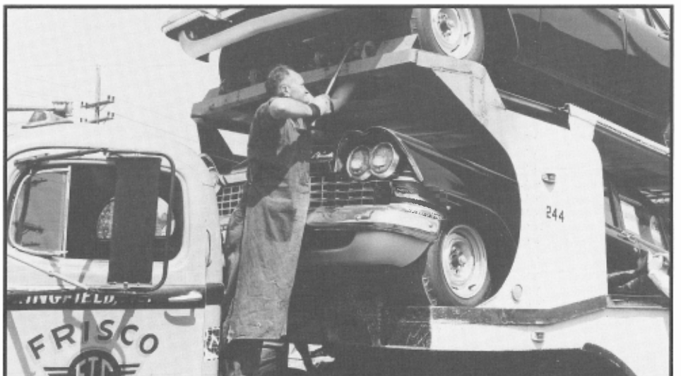
FTC employees make final tie-down checks of autos on transport trailers for shipment via Frisco Piggyback, Fenton, MO, April, 1955. Frisco photo
