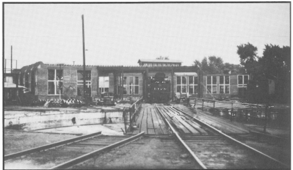
Ft. Smith Roundhouse under construction, July 26, 1945. Frisco photo
