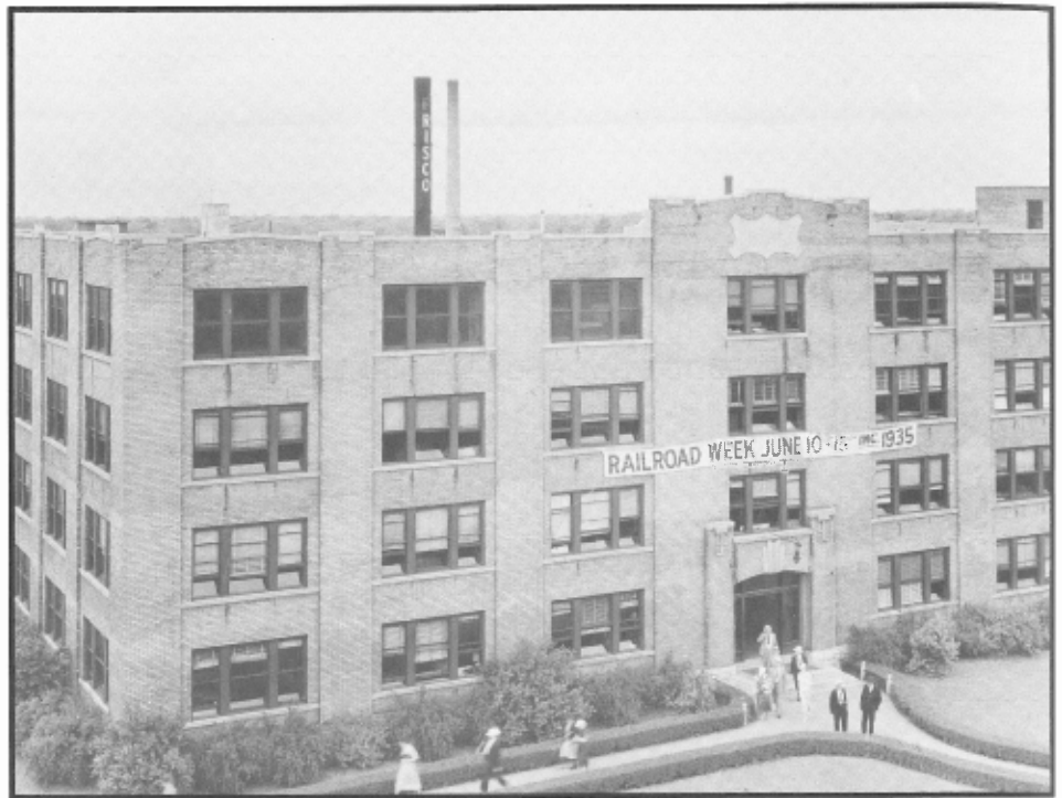
Frisco Office Building, Springfield, MO, June 13, 1935. Frisco photo
