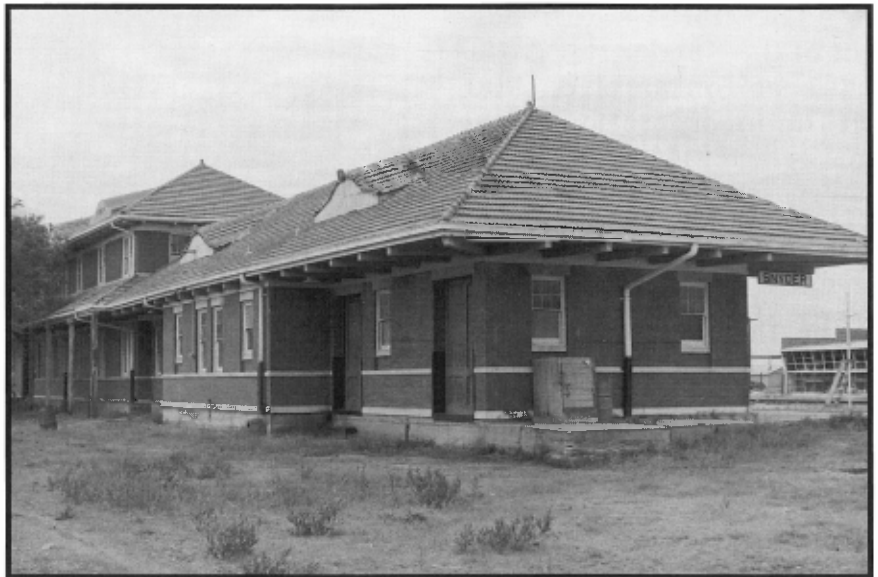
Snyder, OK, depot end, looking northwest. December, 1967
