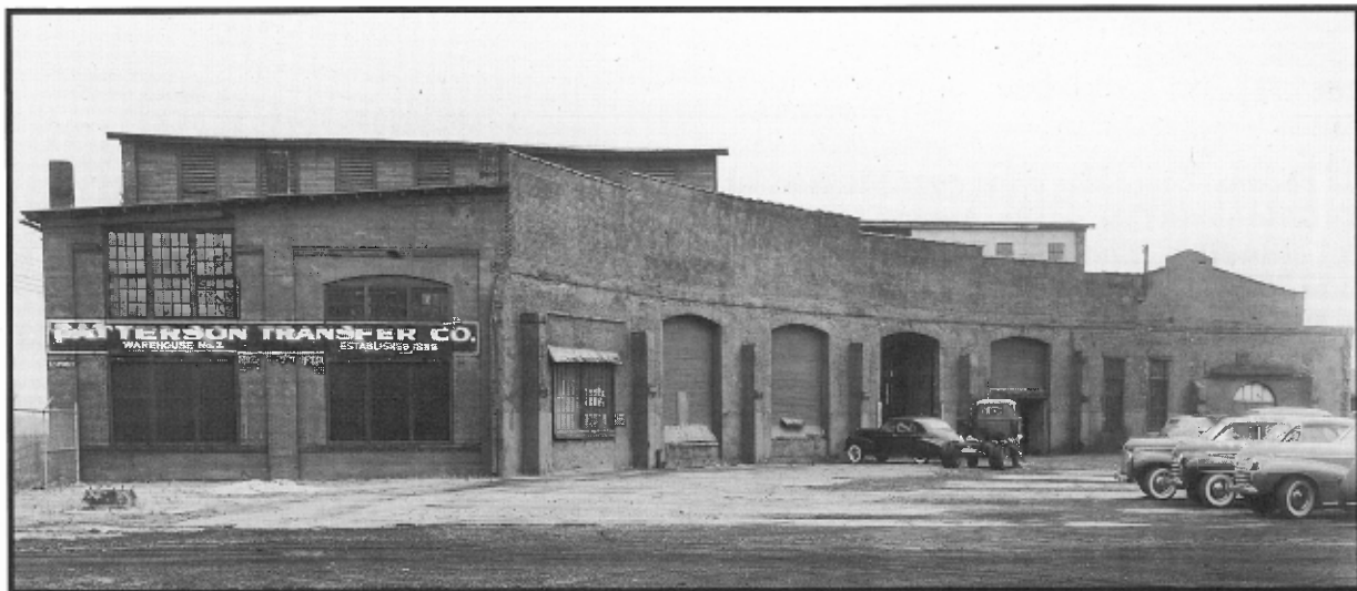
Old Yale (Memphis) Roundhouse, May 27, 1940. south elevation. Frisco photo
