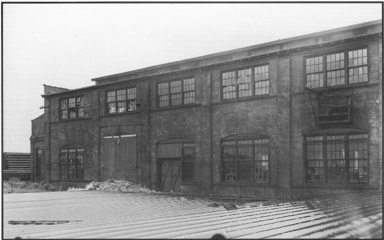
Old Yale (Memphis) Roundhouse, May 27, 1940, north elevation. Frisco photo
