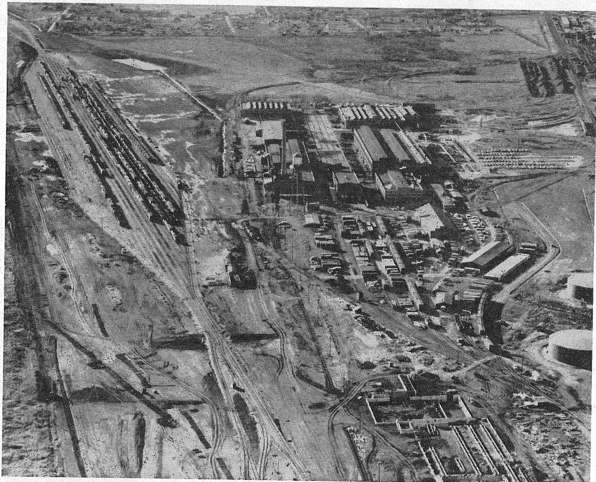
This aerial view of the Springfield yard project, looking toward the West from a point over the juncture of the high-line and the old freight main, shows the progress of the work on the yards and new mechanical facilities.
