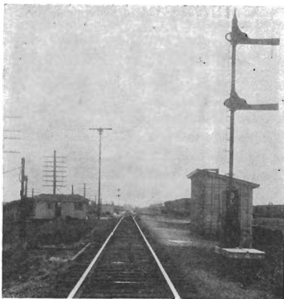
The above photograph is of a two-arm signal at Harvard, Ark., where trains are handled by signal indication only and no written orders issued.
